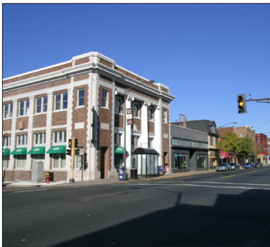
The scale and texture of the older commercial district
