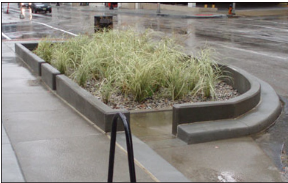
Bioswales to retain and treat stormwater runoff
