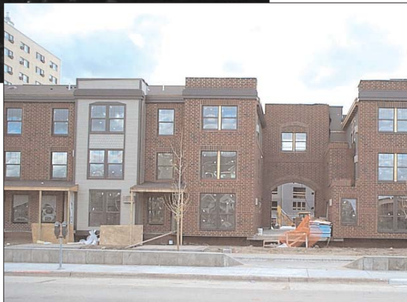
East Village housing under construction
