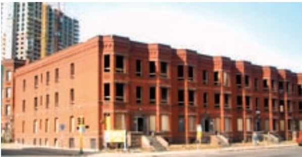
The Lenox condominiums under restoration
