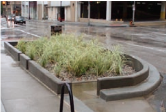
bio-swales to capture and filter rainwater
