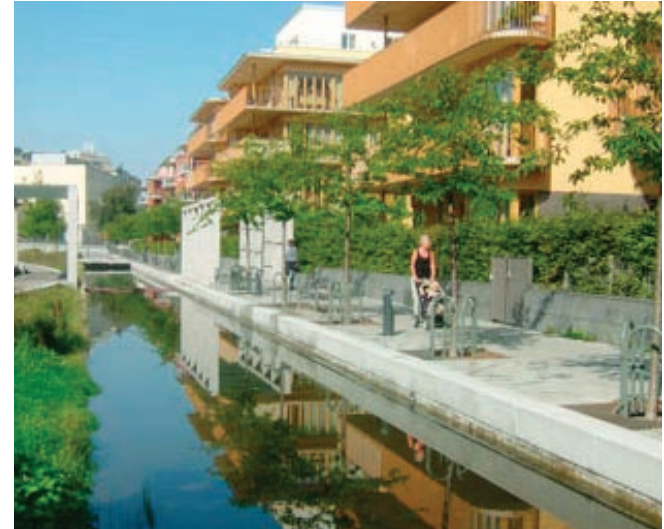
ponds for water recycling
