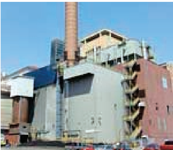
district energy - St. Paul District Heating Plant
