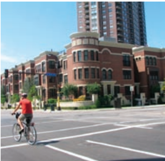
housing liner on Grant Park garage
