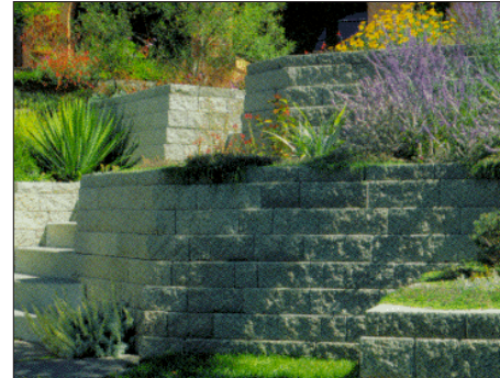
Concrete block modular system - use straight face block only to match existing limestone walls in the area.
