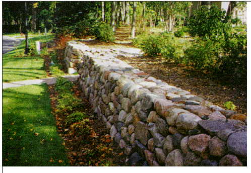
Dry-laid fieldstone wall. Boulders should range from 6" - 18" diameter.
