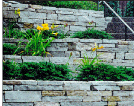
Dry-laid limestone wall. Stone widths vary from 4" - 8".
